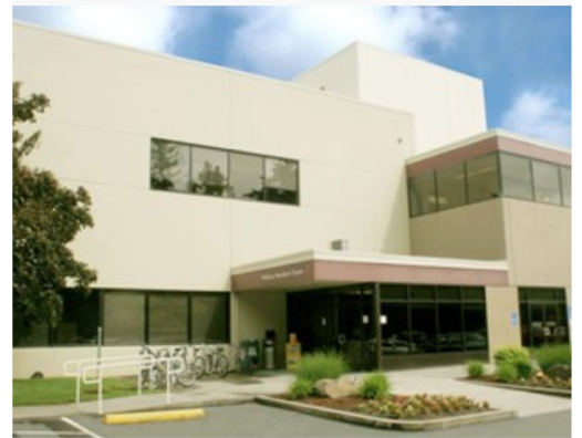
18700 NW Walker Road in Hillsboro, Ore.
